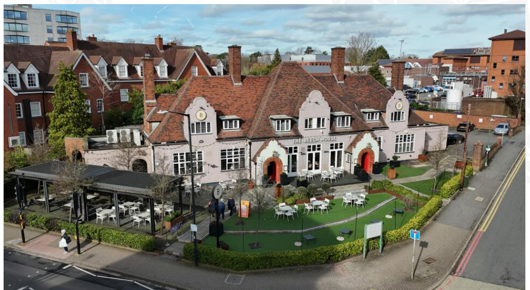
Beech House: Solihull, UK
